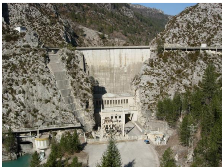
Barrage de Chaudanne (C. GUIN)
