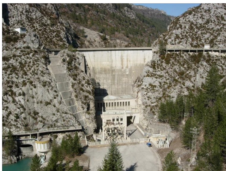
Barrage de Chaudanne (C. GUIN)
